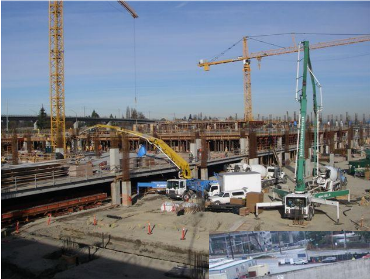
DECK 2, 3, AND 4 PLACEMENT PROGRESS OVERVIEW
