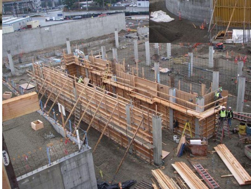
QTA #1 COLUMN & CAR WASH BAY WALL INSTALLATION PROGRESS
